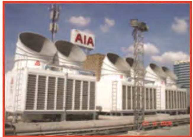
CROSSFLOW TYPE CMS - 500 x 3 SETS AIA TOWER
